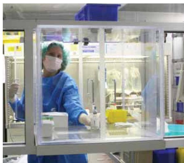
Large pass-through chambers are well suited to MBMC's high compounding volume.
