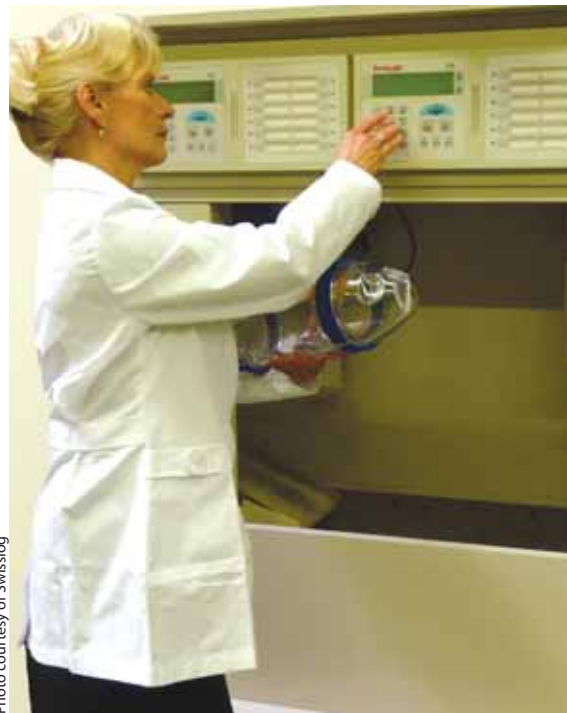
Pharmacy can send urgent medications or first doses, as well as orders for therapeutic substitutions, to the nursing units using pneumatic tube systems.
